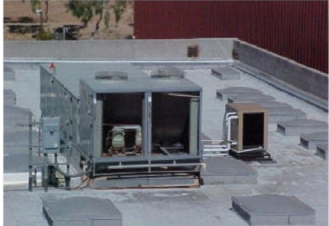
Unit # 3 Trane 20 Ton Capacity
